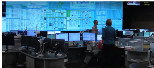
ERCOT control room Source: ERCOT
